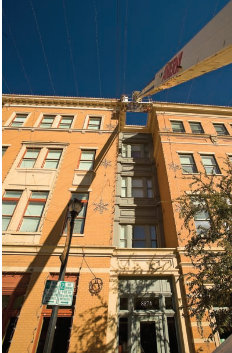
Installing lights at Frisco Square
