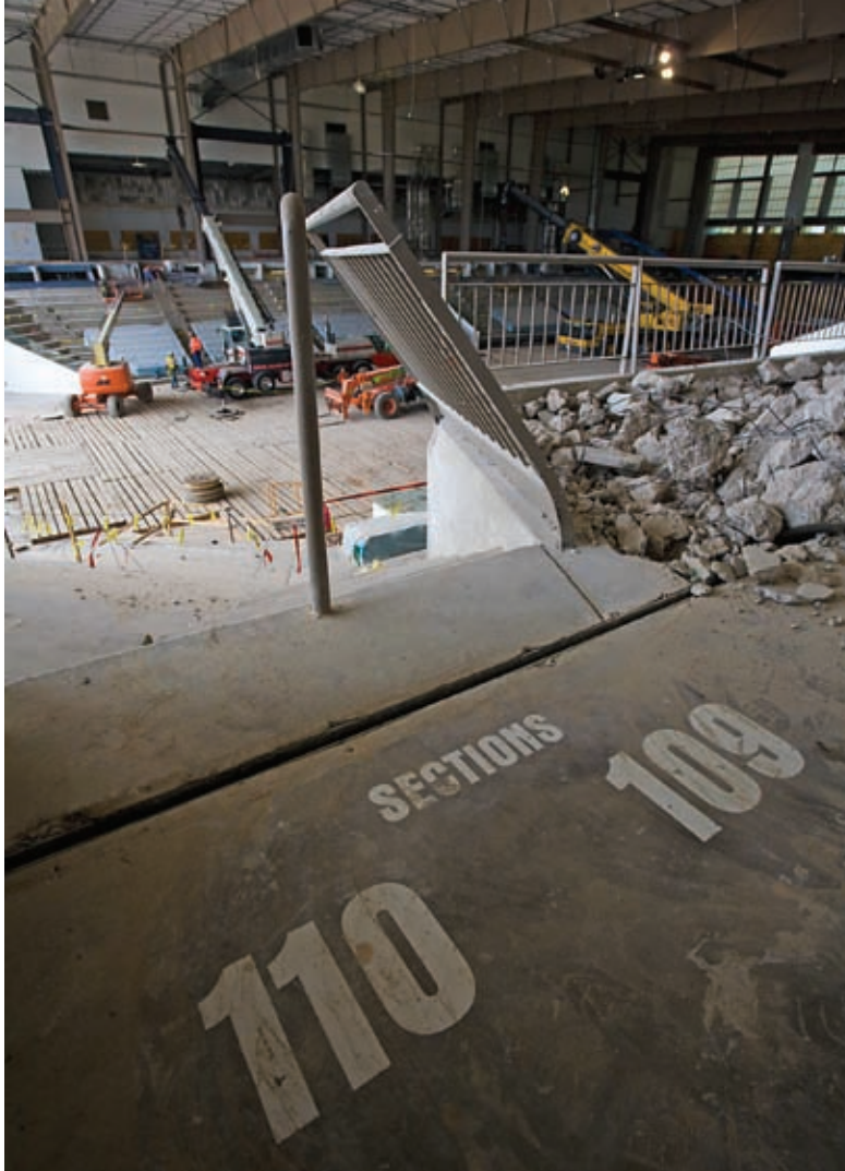
Dr Pepper StarCenter arena interior construction
