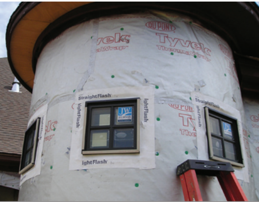
Well sealed window facing north or south save energy photo provided by Green Built Parade of Homes
