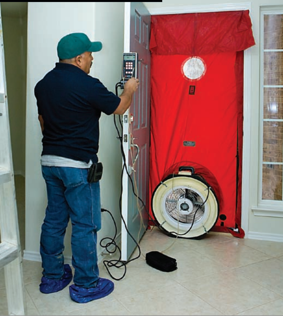
"Blower door" checks detect where air and moisture are getting in and out of a house photo by Chris Fritchie
