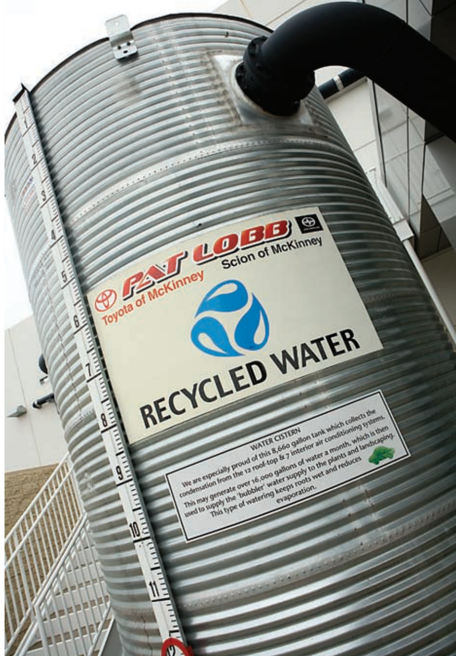
Even the restrooms at Pat Lobb's Toyota dealership tout cutting-edge eco-friendly technology. (far left); Recycling rubber from old tires (center); Air conditioning condensation and rainwater are captured for future use. (right) photos by Chris Frichie
