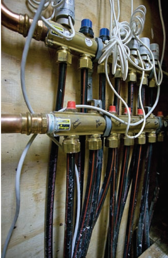
High tech tubing eliminates the need for much of the copper used in new home construction. (left); Bamboo floors and oak doors are part of the eco-friendly design. (right)
