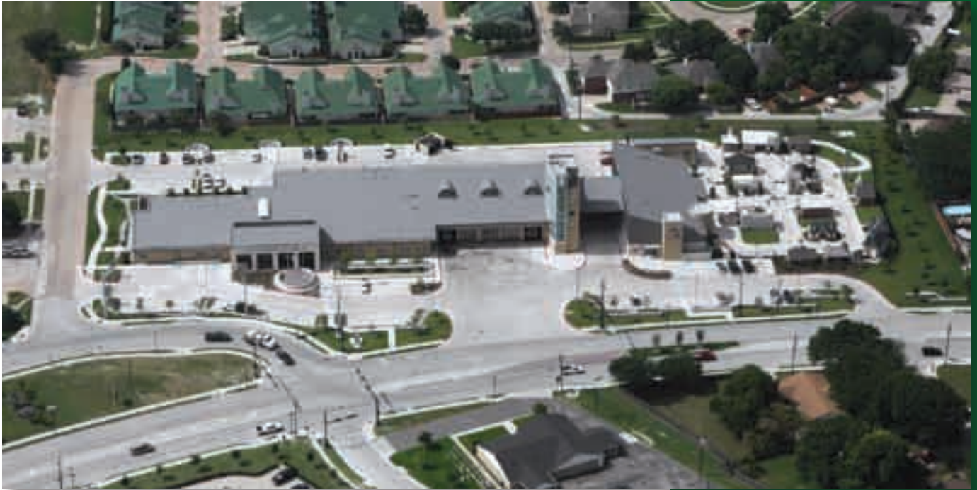
Aerial shot of Frisco Central Fire Station photo by Chris Frichie
