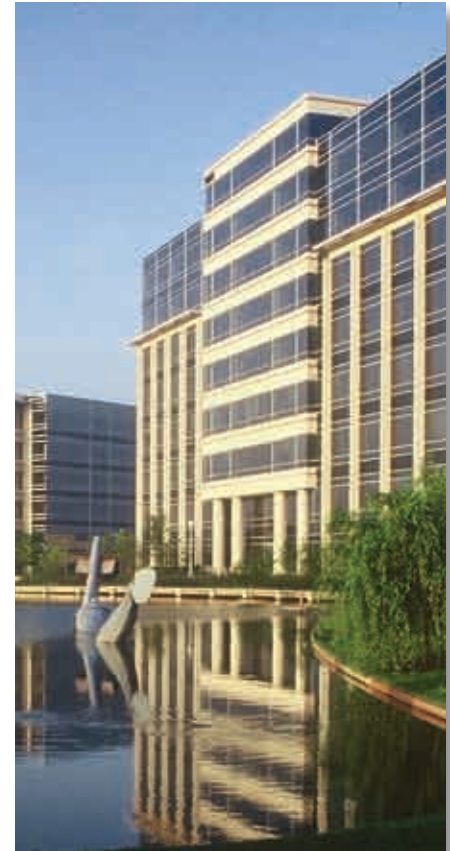
Hall Office Park photo provided by Hall Office Park
