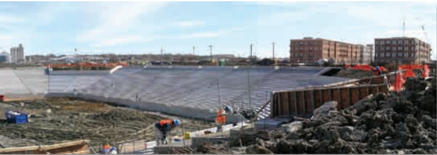
Soccer Stadium Construction, above photo by Chris Johnson
